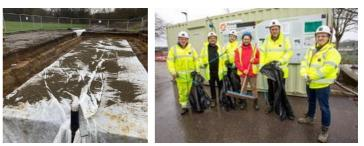
The foundations for the new leisure centre extension are nearing completion and we are now on with the surface water and foul drainage to the building. ISG recently completed the surface water drainage installation from inside the site boundary down to the Red Lion brook, this surface water drainage is attenuated which will slow the release of the surface water into the brook at a reduced flow rate.
